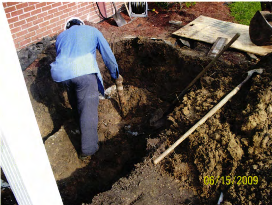
Picture 1: UST 1072Heather during removal. Note concrete slab on top of tank.
