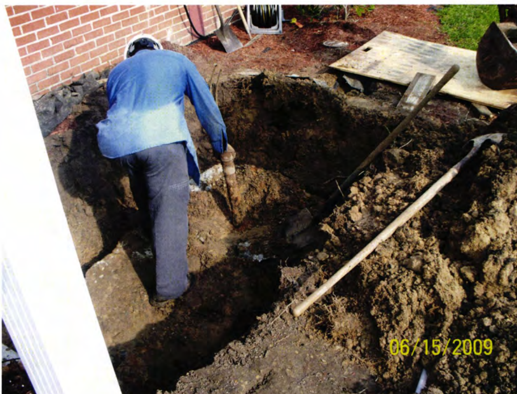
Picture 1: UST 1072Heather during removal.
