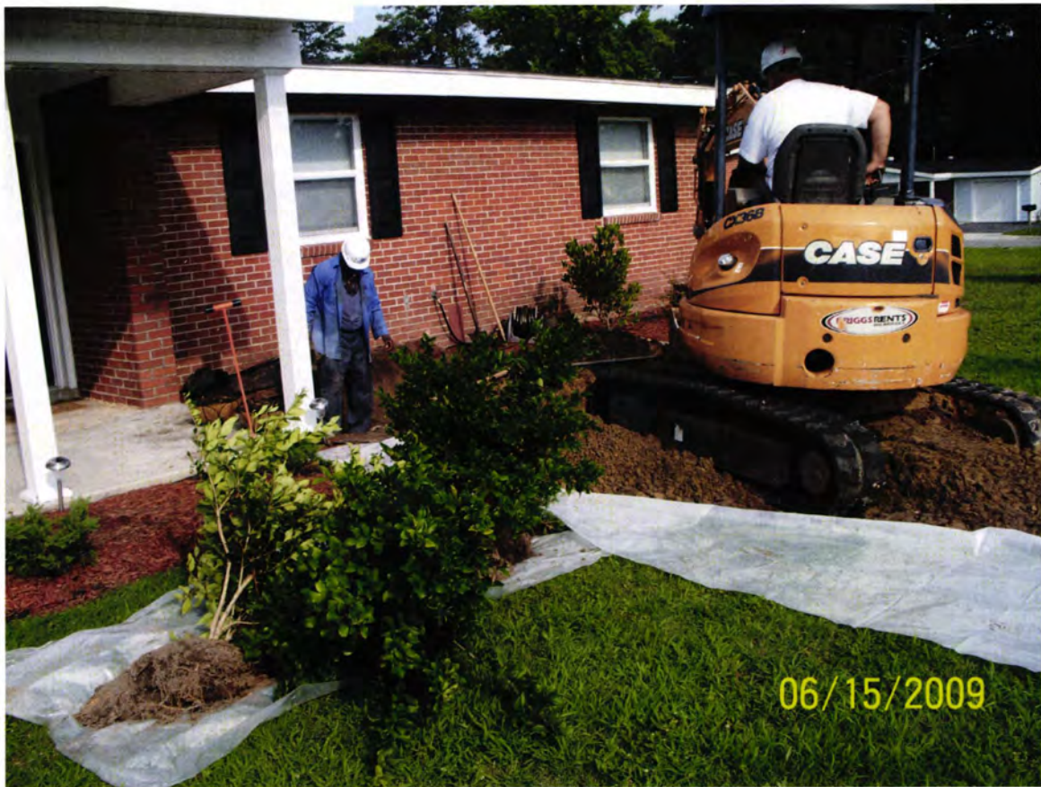
Picture 1: UST 1072Heather site during excavation.
